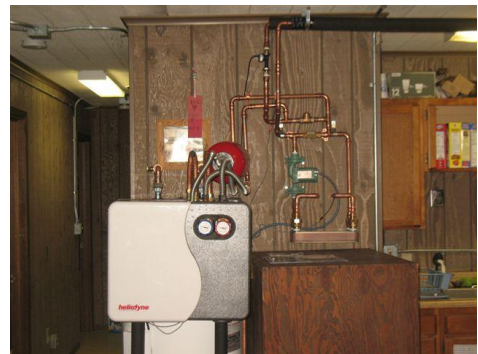
Pro-lite controller and Hilio-pack pro heat exchanger with Wi-Fi and data logging. (insulated cover)
