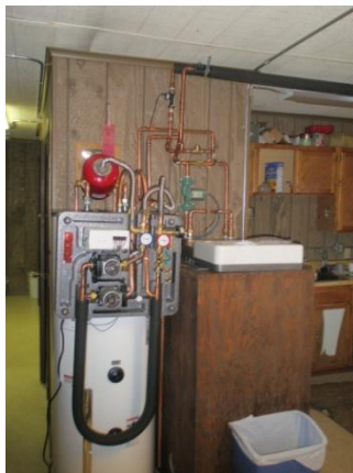
Pro-lite controller and Hilio-pack pro heat exchanger with Wi-Fi and data logging. (uncovered)
