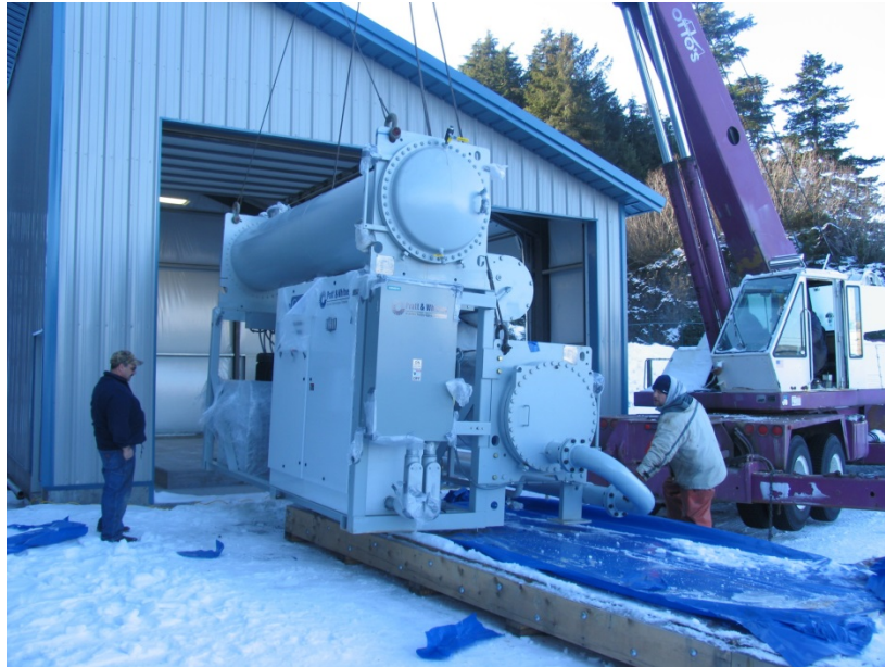
Figure 2: PureCycle 280 Being Installed
