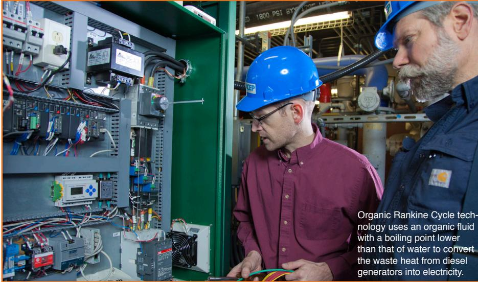
Organic Rankine Cycle technology uses an organic fluid with a boiling point lower than that of water to convert the waste heat from diesel generators into electricity.
